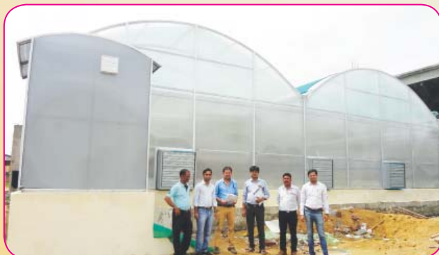
Newly installed Green House at GBP's permanent site
